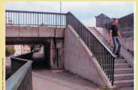
Above: a bridge in Toulouse with a triple ramp: access to the bridge to cross to the opposite side, route passes under the bridge ensuring continuity along the bank of the Garonne and access from the road; below: the same bridge viewed from the other side, with stairs providing direct access for pedestrians, instead of the detour via the ramp (note the concrete stair «ramp» for bicycles or pushchairs; alternative solution alternative: a single wheeling channel for users carrying a bicycle or a double channel for bicycles and pushchairs)
