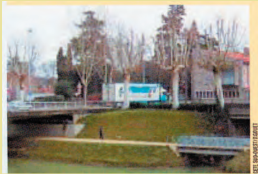
Path along the banks of the Gers, with railings at certain points where it is particularly dangerous (narrow path crossing a structure)
