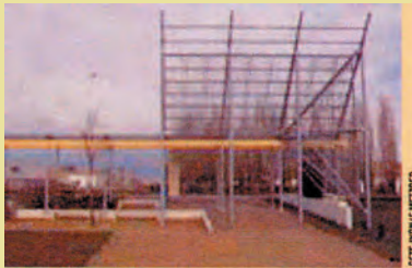
Modern footbridge in an industrial zone (along the bank of the River Gers)
