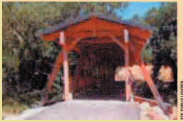
Covered footbridge on cycle touring route built by the Luberon regional nature park and crossing the River Largue near Manosque
