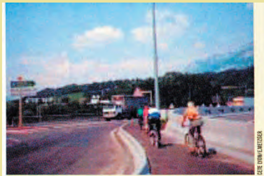
Road bridge in Chambéry where the lanes have been narrowed – thereby reducing the speed of motorised traffic – by constructing a path for pedestrians, cyclists and PRMs, of benefit to all users; cyclists can ride either on the road or within this safety zone
